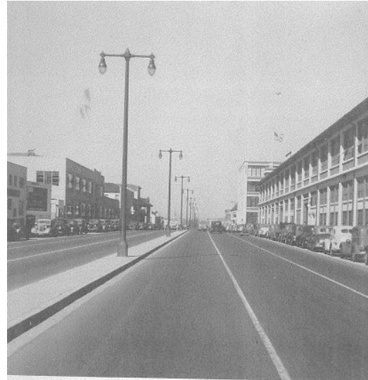
1942- Third Street Reconstruction
