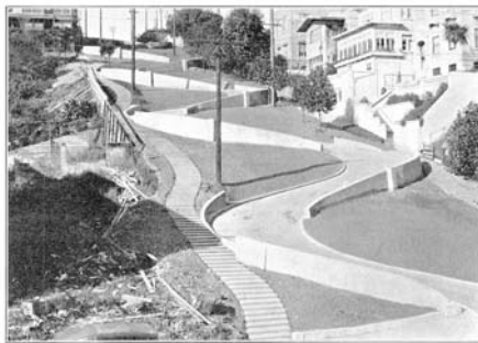
LOMBARD STREET, LEAVENWORTH STREET TO HYDE STREET Winding roadway on brick pavers and 20% rubble concrete pavement.
